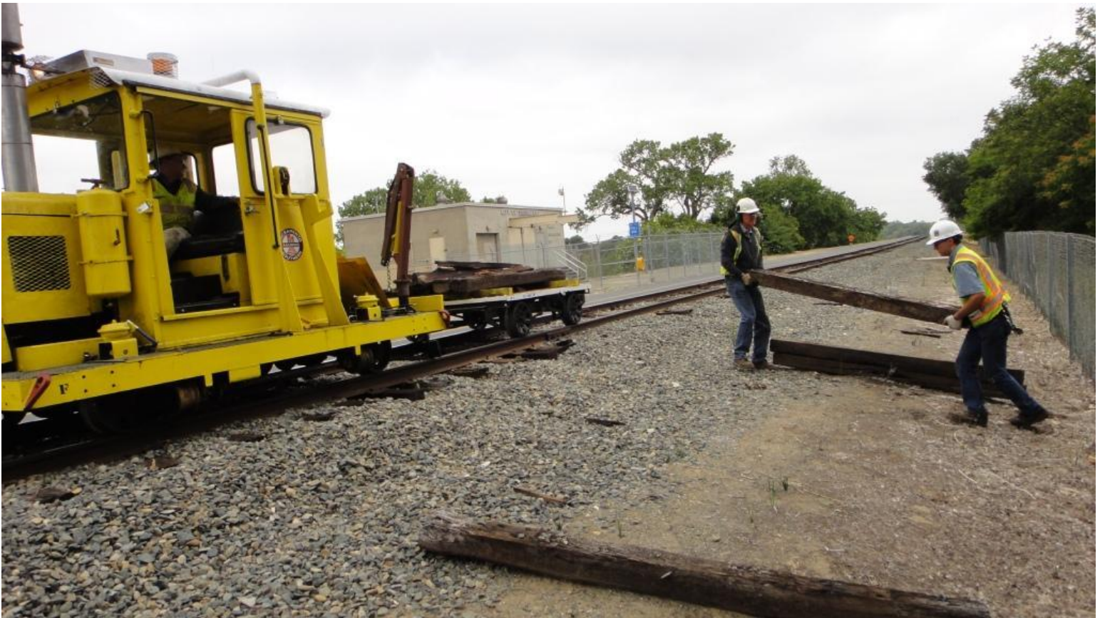
Mike H. pilots the Kalamazoo tug while Steve and Matt load dead ties south of MP 2.5 onto a flatcar for disposal
