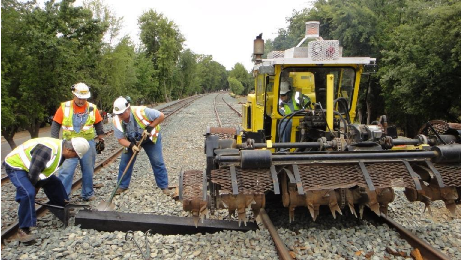
Heather operates the inserter function of the scarifier. Chris tries to dig out from under the tie to prevent it from going in at downward angle. John guides the scarifier's inserter grapple to keep it straight.
