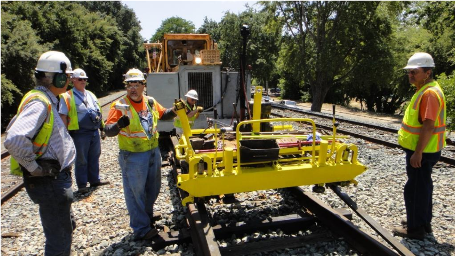
Mike F. flaunts "Maxwell's Silver Hammer" as the rail-lifter is deployed...
