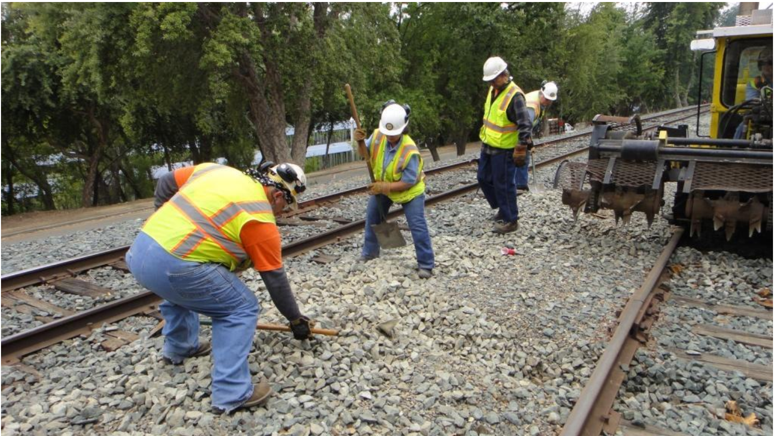
There was a whole heck of a lot of digging that needed doing as Mike F. and Pam can attest...
