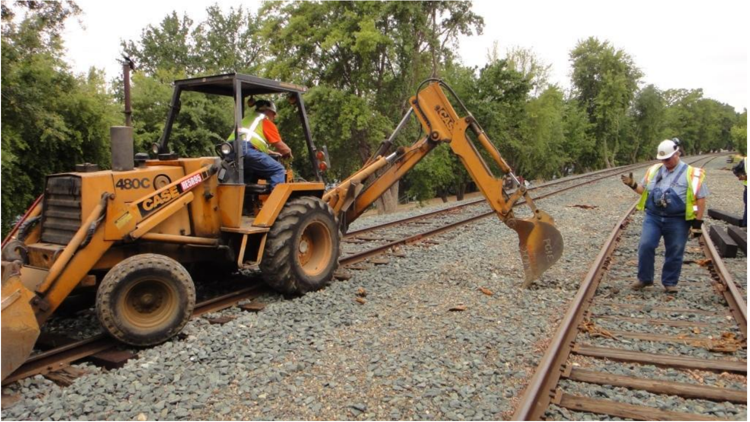
Chris guides Harry on the back-hoe who was digging out a trench in which a tie could be placed for insertion on the siding
