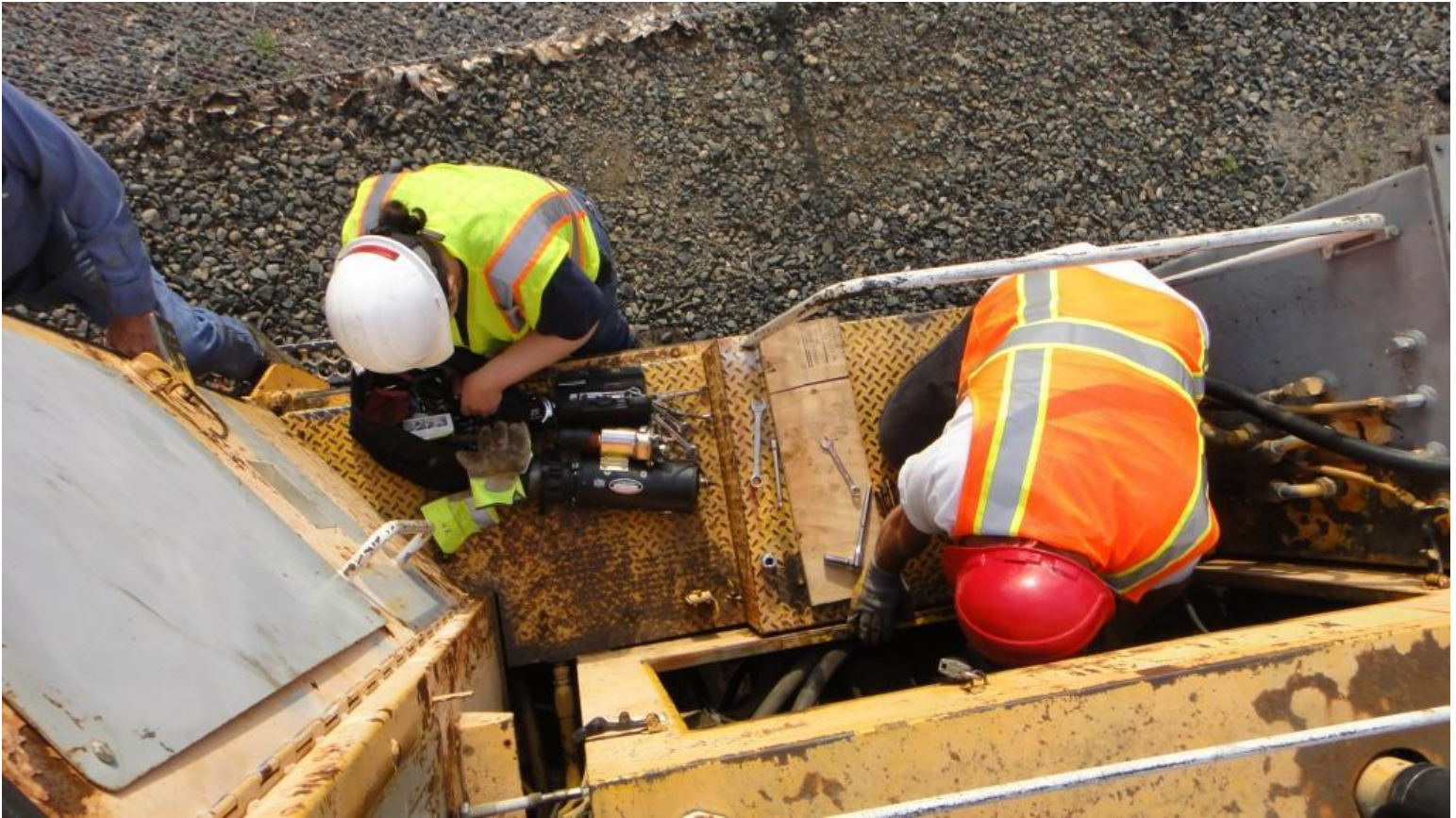
Heather and Joe prepare to install a new starter-motor and solenoid in the old-old tamper
