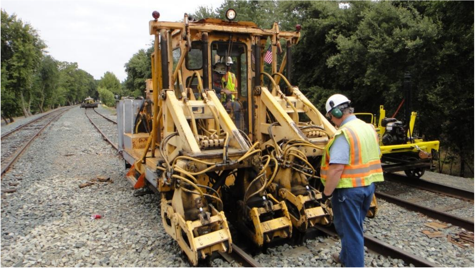
After the new ties are inserted, they are tamped-up against the base of the rails. Chris guides Mike F. in the tamper.
