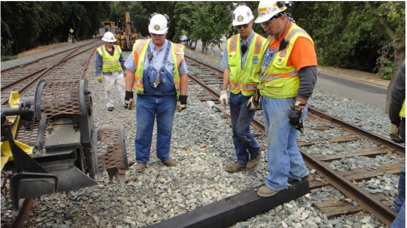
Mike F. tries stomping down on the tie to reduce the angle of insertion.
