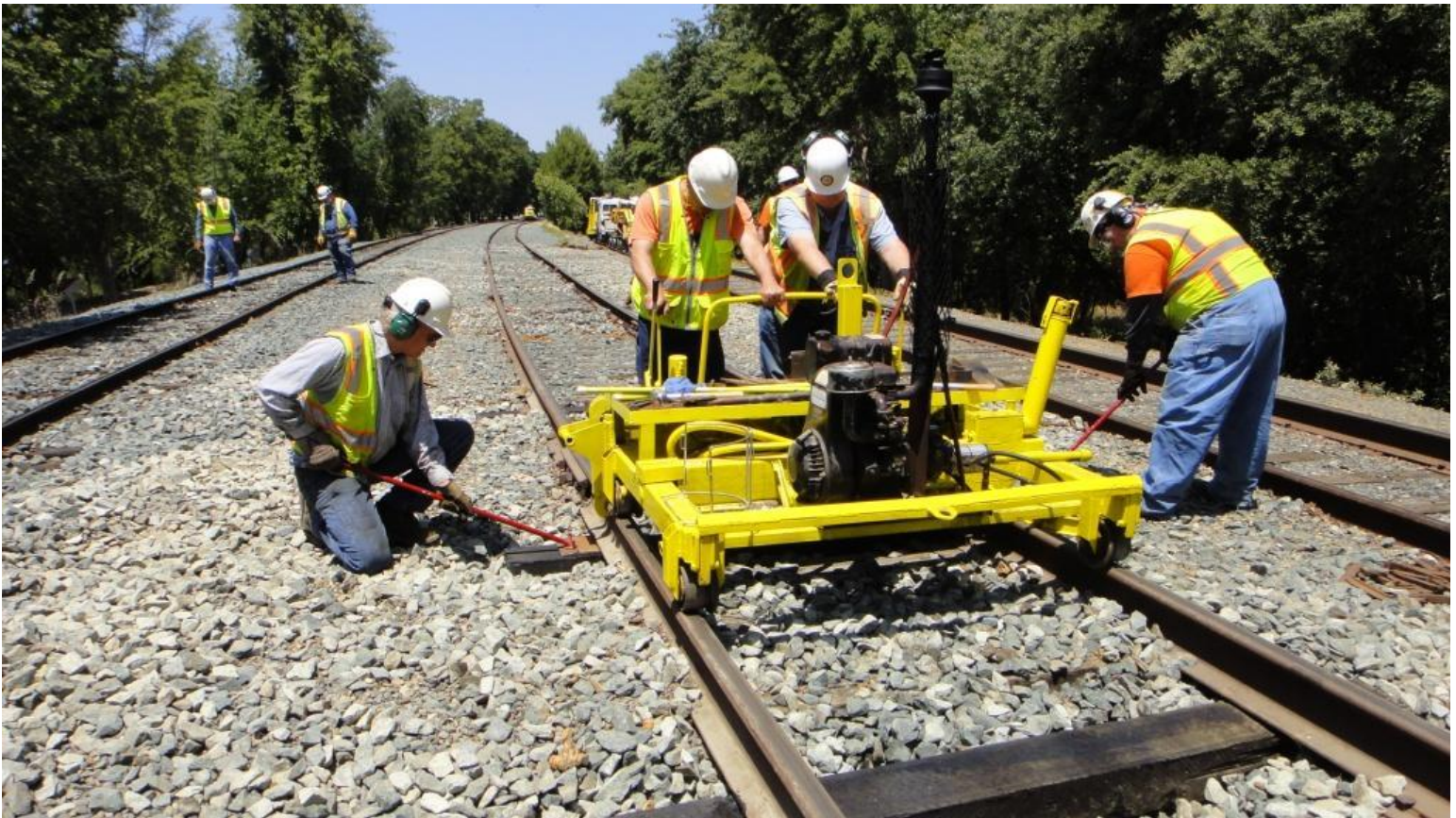
Steve and Mike F. use specially made wands to insert the double-shouldered tie-plates as John and Chris operate the rail-lifter
